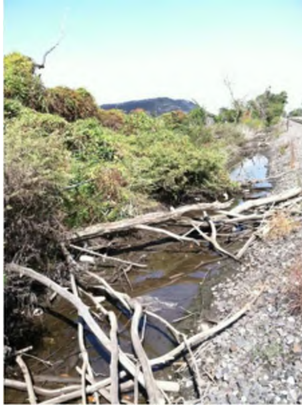
Photo 3: Drainage ditch WCC-B looking north (September 2013).
