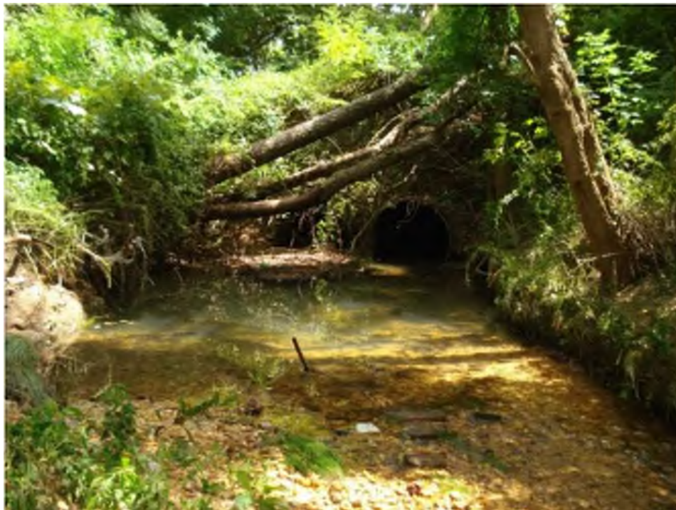
Photo 42: Wetland WGO-A looking east towards culvert in Chestnut Branch (August 2013).
