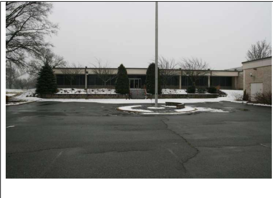
Photograph 7: Northwest elevation (façade) entrance of Block B. Note Block A is visible on the right. Looking southeast (January 2019).
