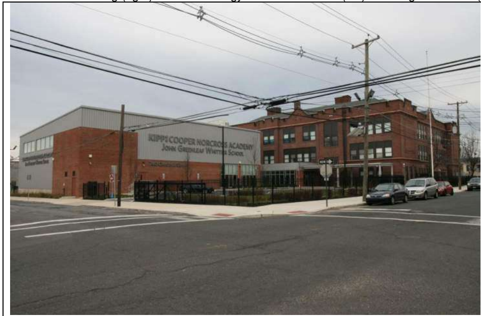
Photograph 1: Overview of the John G. Whittier School at 740 Chestnut Street, showing the east (side) and north (front) elevations of the 1910-11 main building (right) and the 2017 gymnasium addition (left). Looking southwest (December 2018).
