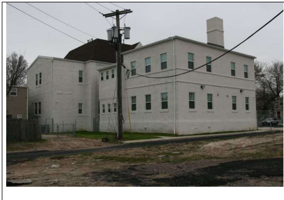
Photograph 4: East (side) and north (rear) elevations. The original (1888 to 1889) building is visible at left, the circa -1900 rear addition is shown at right, and one of the two circa -1994 additions is visible in the center. Looking southwest (December 2018).
