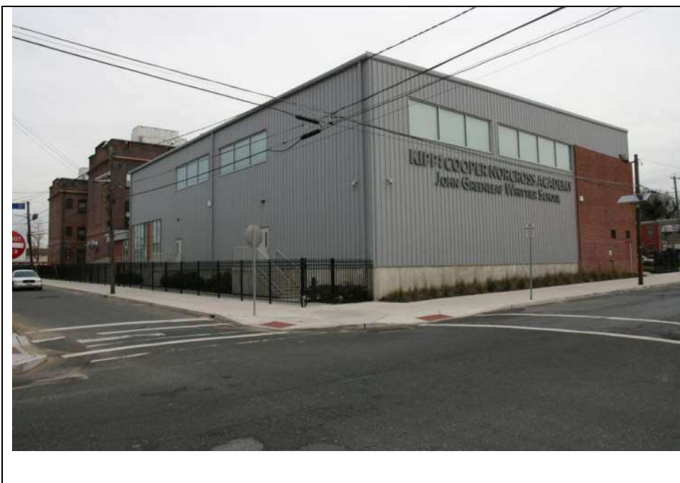
Photograph 13: South (rear) and east (side) elevations of the 2017 gymnasium, looking northwest (December 2018).
