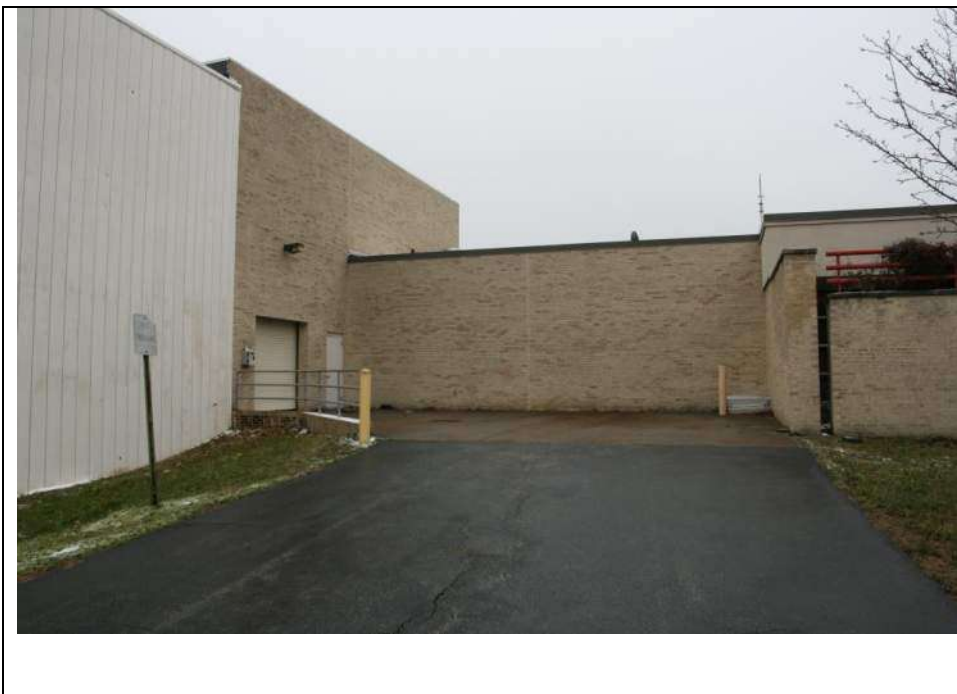
Photograph 19: Northeast (side) elevation of Block D on the right, note Block E's northeast (side) elevation and Block A's southeast (front) elevation are also visible to the left and right respectively. Looking northwest (January 2019).
