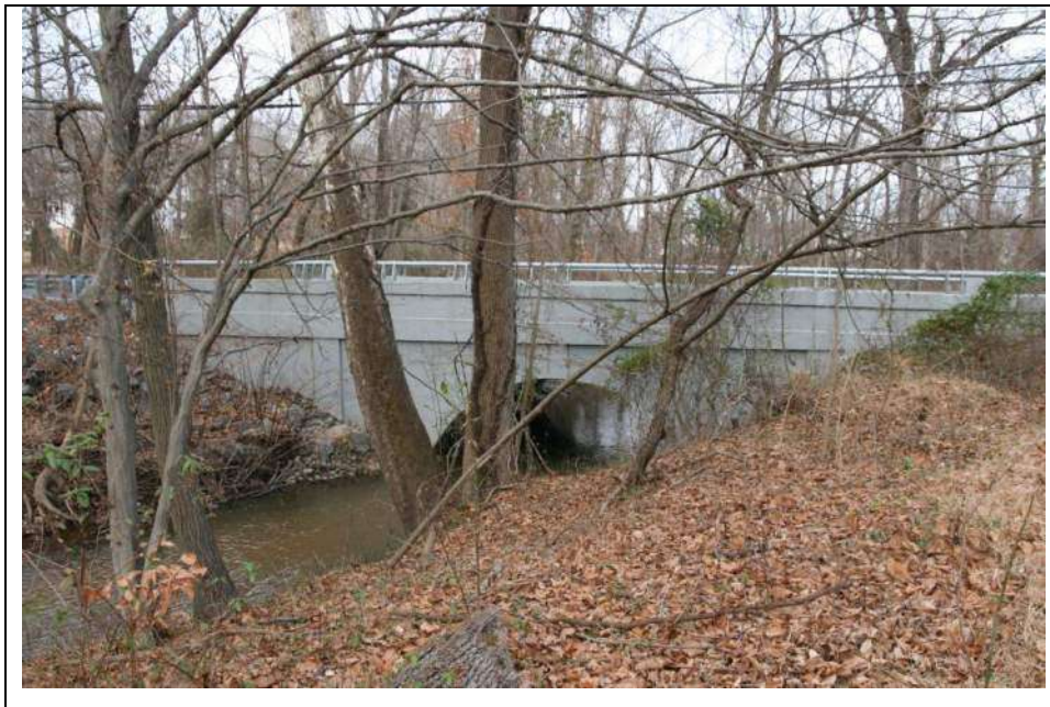
Photograph 7: South (upstream) elevation. Looking northwest (December 2018).
