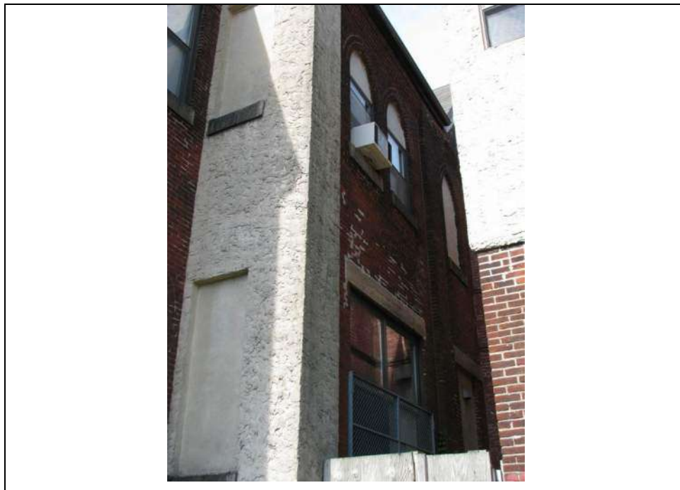
Photograph 5: Partial view of the east (side) and north (rear) elevations of the original 1888 to 1889 building. Looking southwest (May 2014).
