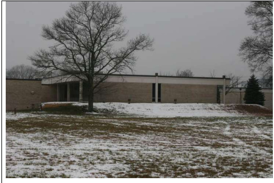
Photograph 6: Northeast elevation (side) of Block B. Block F is visible on the left. Looking southwest (January 2019).
