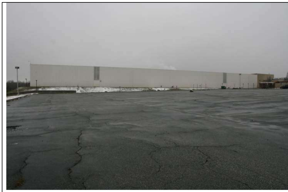
Photograph 21: Northeast elevation (side) of Block E and upper parking lot. Note the northeast elevation of block D is visible on the right. Looking southwest (January 2019).
