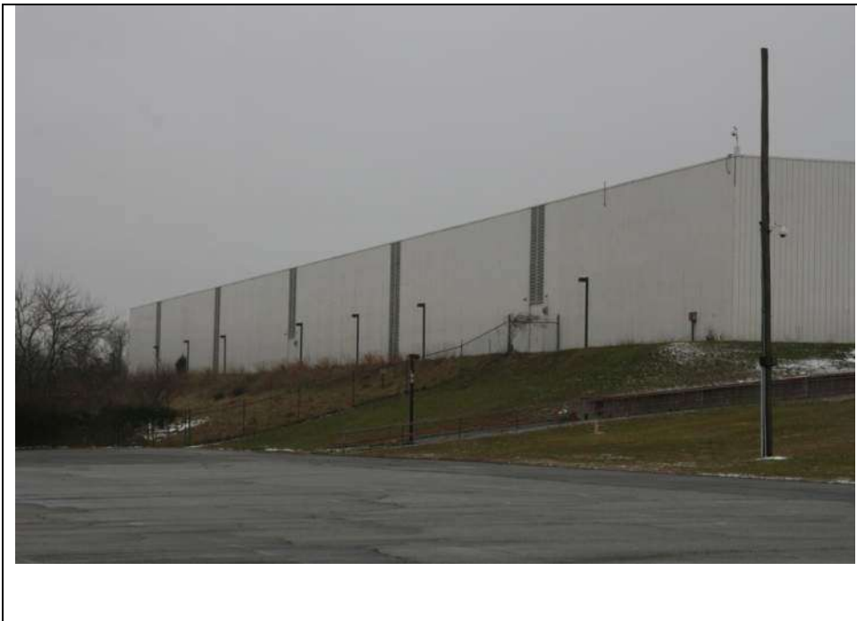
Photograph 20: Southeast (front) and northeast (side) elevation of Block E and lower parking lot. Looking northwest (January 2019).
