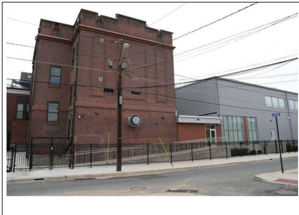
Photograph 8: South (rear) elevation of the eastern 1922 rear classroom wing (left). A portion of the 2017 gymnasium addition is visible at the right-foreground. Looking northeast (December 2018).
