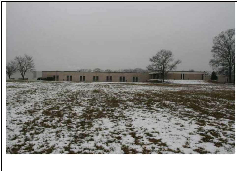
Photograph 5: Northeast elevation (side) of Blocks F on the left and Block B on the right. Note Block E is visible on the far left. Looking southwest (January 2019).
