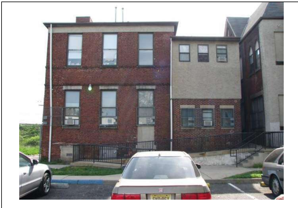
Photograph 3: West elevations of the circa -1900 rear addition (left) and one of the two circa -1994 additions (right). The north (rear) elevation of the original 1888-89 building is partially visible as well (far right). Looking east (May 2014).
