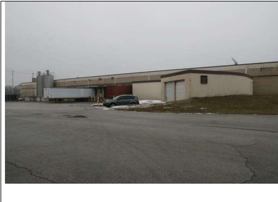
Photograph 16: Southwest elevation of Block C. Looking northeast (January 2019).
