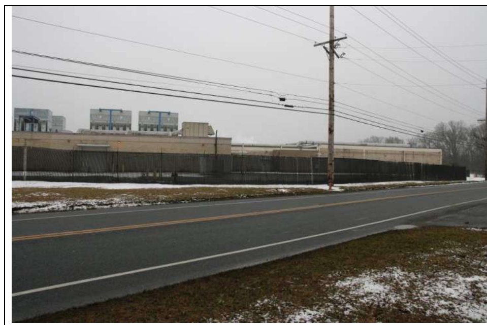
Photograph 13: Northwest elevation of Blocks G on the left, A in the center, and C on the right. Looking southeast (January 2019).
