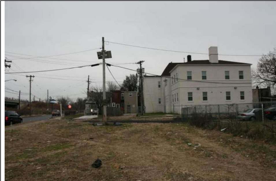
Photograph 9: Overview showing the Jesse W. Starr School in context. Looking south toward the rear of the property (December 2018).
