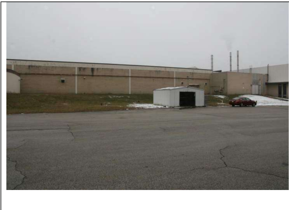
Photograph 17: Southwest elevation of Block C on the left, D on the far right, and outbuilding I. Looking southeast (January 2019).
