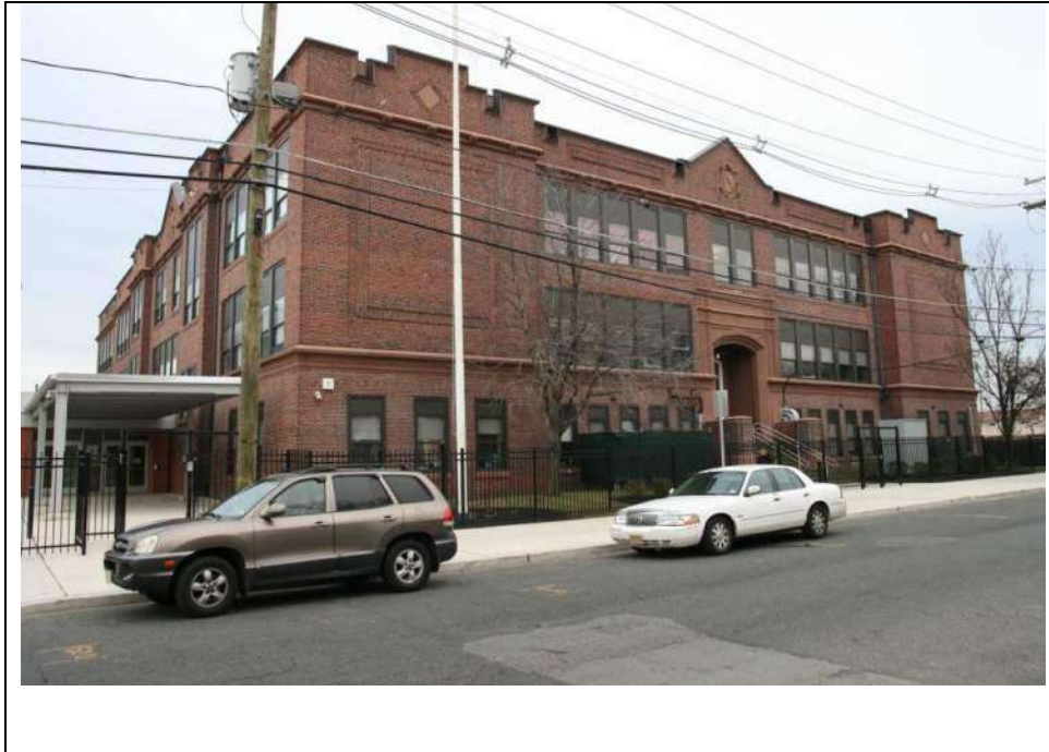
Photograph 2: East (side) and north (façade) elevations of the original 1910-11 section of the John G. Whittier School at 740 Chestnut Street, looking southwest (December 2018).
