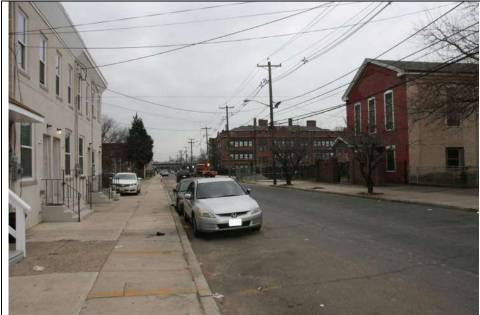
Photograph 14: Overview of the John G. Whittier School in context, looking east along Chestnut Street (December 2018).
