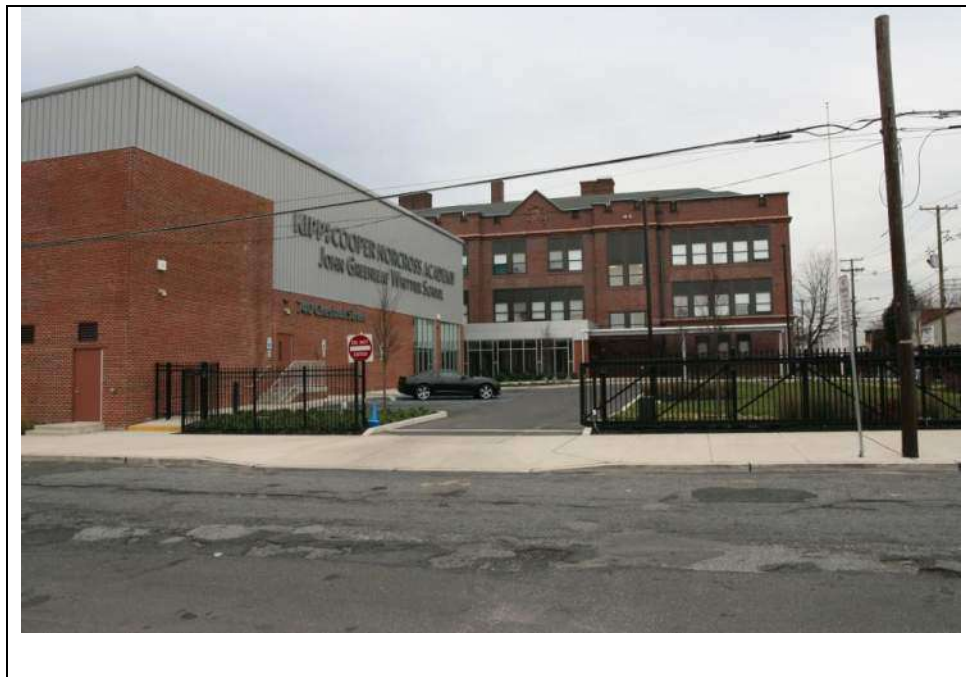
Photograph 5: East (side) elevation of the original 1910-11 section of the John G. Whittier School, and north elevation of the 2017 gymnasium addition, looking west (December 2018).
